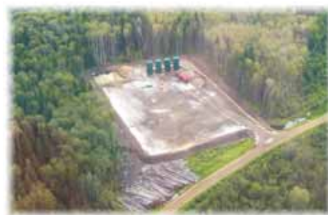
Construction of surface site on Bigstone Cree Nation lands, Alberta.
