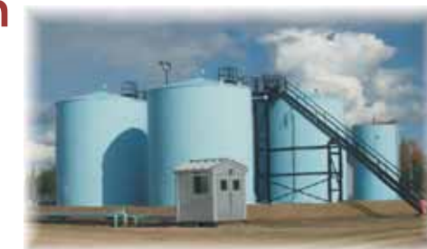
Oil tanks at O'Chiese First Nation, Alberta.
