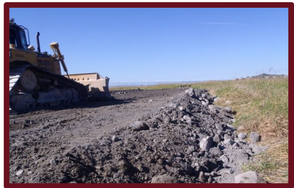
Levelling and packing of fill
