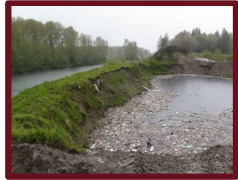
Do not fill near waters that are fish-bearing or that are connected to fish-bearing waters.
