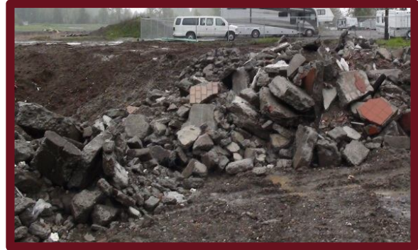
Asphalt and brick demolition waste are not acceptable as fill.
