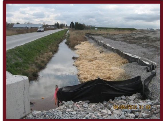
Mulch, a silt fence, and gravel all protect water in a ditch.
