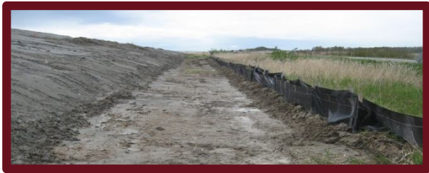
Silt (glacial till) used for a landscape berm
