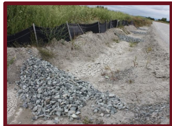
A gravel check-dam in a drainage ditch with a silt fence.
